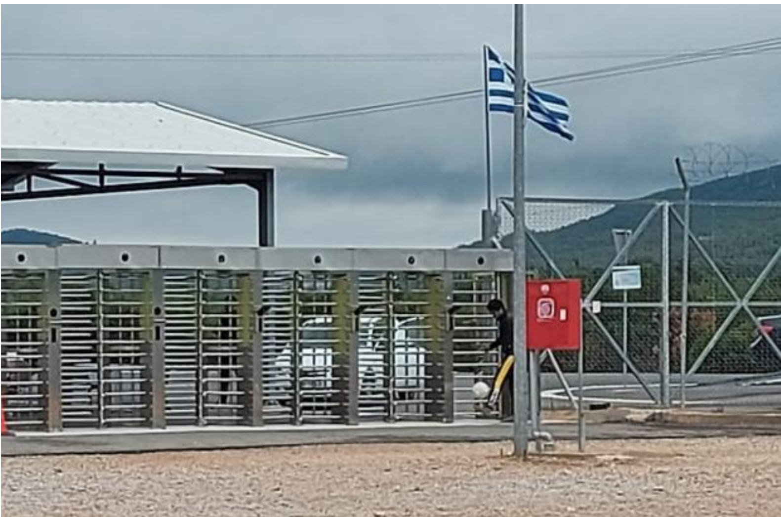
Image of the entrance, the access road, to the newly built Malakasa field considered "closed" in which you can see the multiple security and control systems such as the fence, the smart posts or the barbed wire
